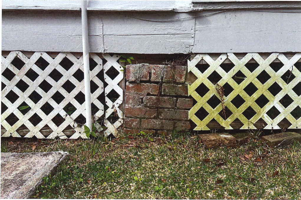
Sinking Pier - East
