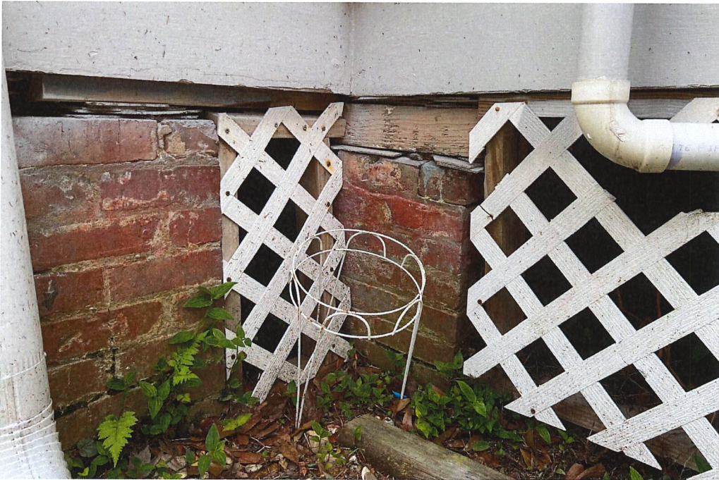
Existing Piers - East
