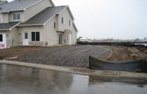
Properly constructed BMP for vehicle tracking.
