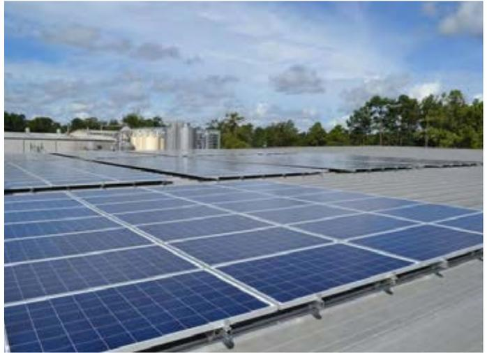
*Abita Brewing Co. installed 340-panel 84 kilowatt photovoltaic rooftop solar system in 2013. The solar power is used to brew beer.*
