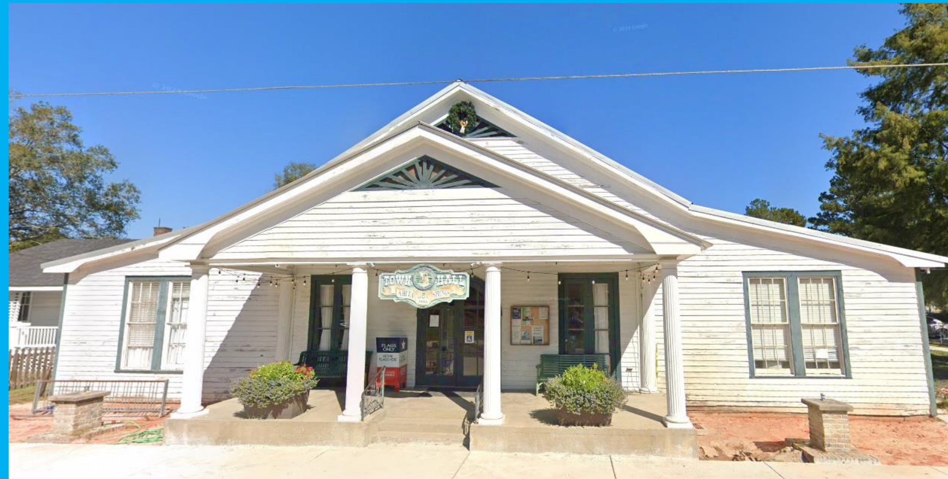
Town Hall – 22161 Level Approximately 6,750 sqft
