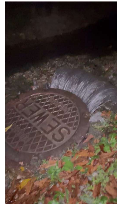
Overflow at Manhole Near 71599/71606 Levenson St
