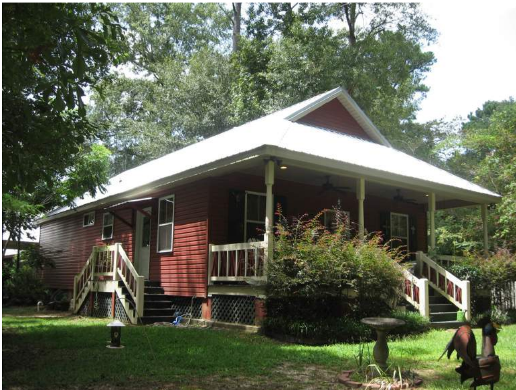
Example of compatible infill construction at 72059 Cypress Street. Designed in a gable front plan, it has appropriately sized windows, a full-width porch and a gable metal roof.
