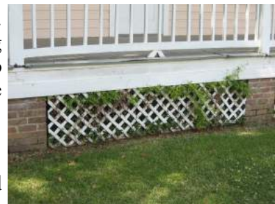
Lattice is an appropriate addition between brick piers (72090 Maple Street).
