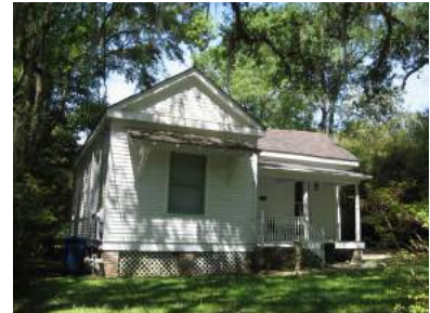
A gabled ell dwelling at 11613 Keller Street.
