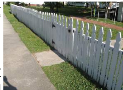
Appropriate height and designed picket fence at 22155 Level Street.
