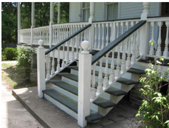
Wood porch elements and stairs should be preserved and maintained (71648 Maple Street).
