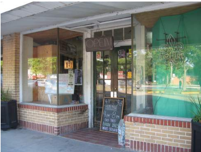
The 1903 Rauch's Grocery (Abita Springs Market ) original storefront has a recessed entrance flanked by display windows on brick bulkheads (22069 Highway 59).
