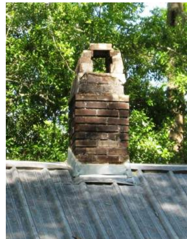
The brick chimney and its cap at 72125 Gum Street is an original feature and should be preserved.
