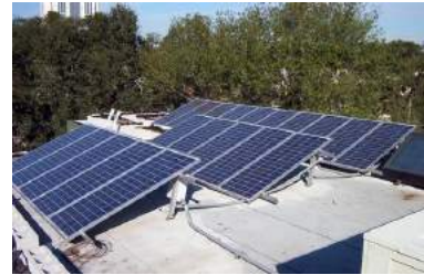
Rooftops are the preferred location for solar panels.
