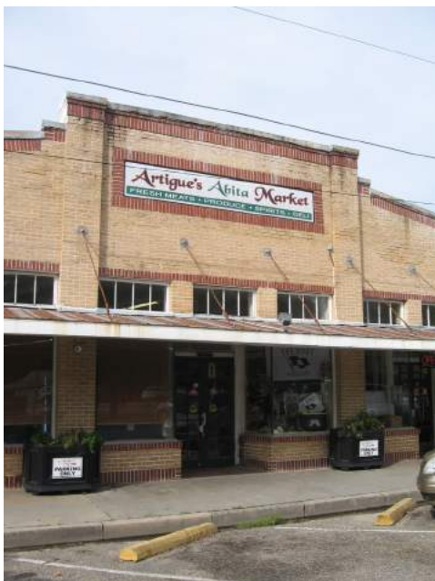
Retain historic awnings like the metal awning spanning the entire façade of the Abita Springs Market (22069 Highway 59).
