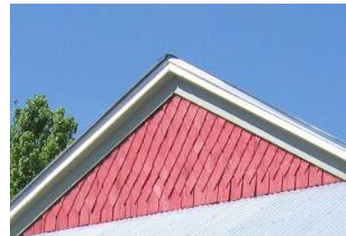
Gable fields are often decorated with sawtooth or fish scale wood shingles (71667 Leveson Street).
