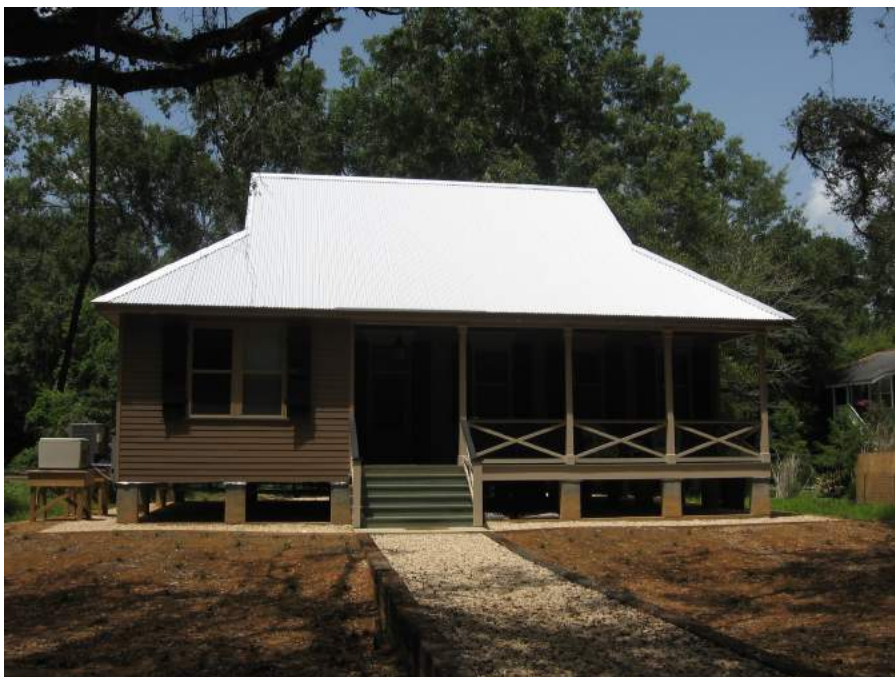
Example of compatible one-story infill construction at 22017 Second Street. The dwelling has a recessed porch, metal roof and pier foundation.
