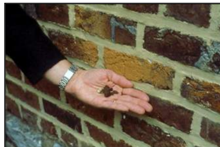
No—Do not use any abrasive cleaning on historic brick walls which could lead to spalling and cracking.
