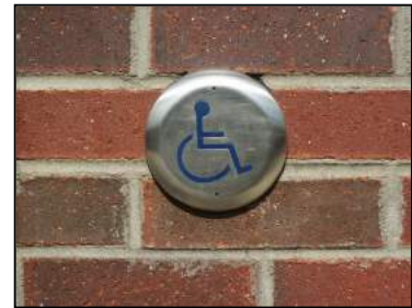
Push plates for ADA access are appropriate solutions for access into commercial buildings.
