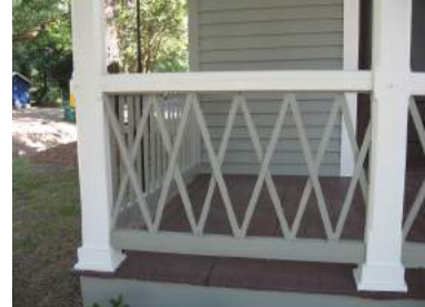
Appropriate rebuilt railing at 22179 Main Street.
