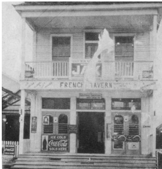
Historic photographs of Abita Springs commercial buildings provide templates for new construction including first floor galleries and second story balconies (Photos courtesy http://tammanyfamily.blogspot.com/2016/06/old-photographs-of-abita-springs.html ).
