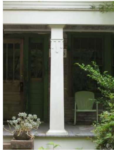
When wooden elements like porch columns require repair or replacement, they should be rebuilt to match their original design or in a style compatible with the style of the dwelling. This Bungalow style column was rebuilt after being damaged by Hurricane Katrina (71446 St. Joseph Street).
