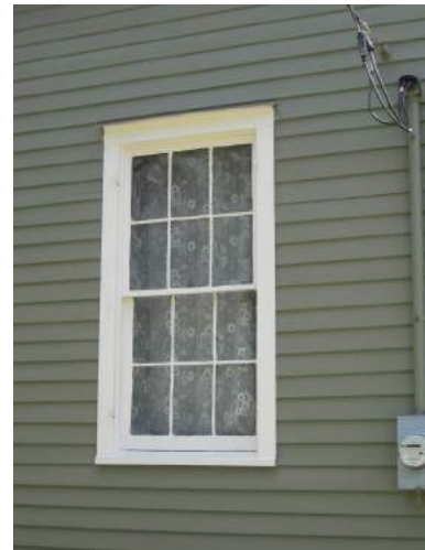
Original six-over-six, wood-sash window at 22222 Level Street.
