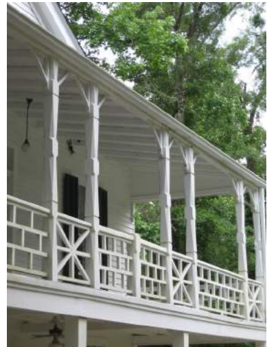
Porches such as at 22128 5th Street have an abundance of wood elements, including milled posts, railing and balusters, and ornamental trim.
