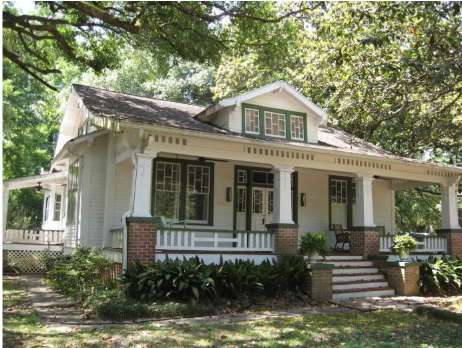
Porches help define a dwelling's style, like this Bungalow's wide porch with tapered posts on brick piers. Porch elements should shall be preserved and maintained (22014 2nd Street).
