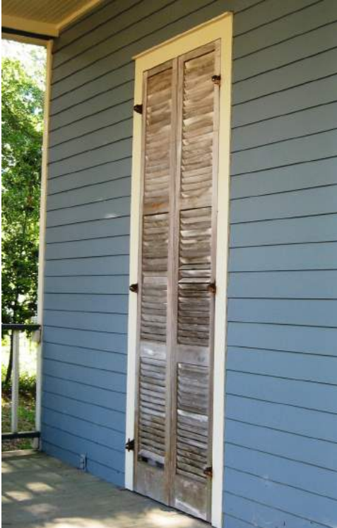
Original window shutters protect the window behind them and these should shall be preserved and maintained.
