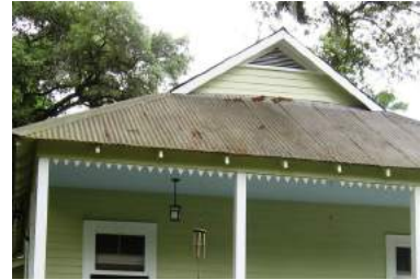
Many houses in the district have crimped metal roofs that contribute to the character of the building (71561 Hickory Street).
