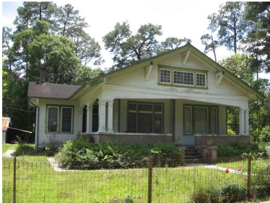
This Bungalow dwelling at 22236 Level Street was built in 1916. Its multi-light windows, wide porch with columns on a closed rail, and eave brackets are character-defining features of this style.
