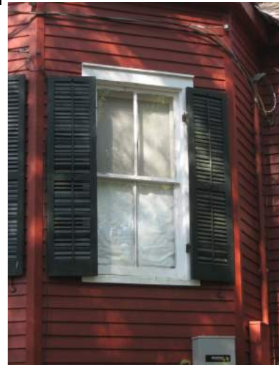
Original window shutters at 22205 Main Street.
