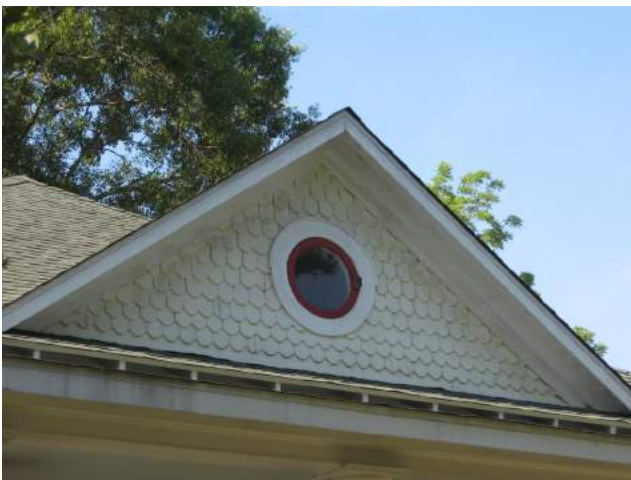
Left: Original wood shingles in the gable field at 22200 Main Street.
