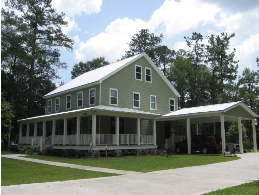
Example of compatible two-story infill construction at 22382 Level Street. The dwelling has a one-story wraparound porch, appropriately sized windows, and gable roof carport.
