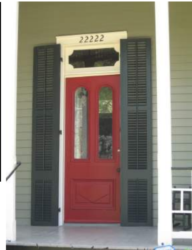
This entrance displays its original door, transom, and wood shutters (22222 Level)
