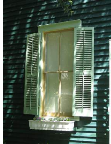
Original two-over-two, wood-sash window with working shutters at 22021 Main Street.
