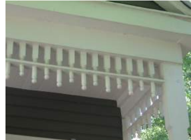
Trim such as this milled wood valance should not be removed or concealed (72170 Gum Street).
