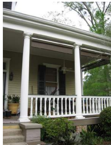
Original porch designs should not be enclosed or altered (22323 Level Street).
