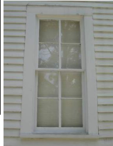
Original four-over-four wood sash windows at 71648 Maple Street.
