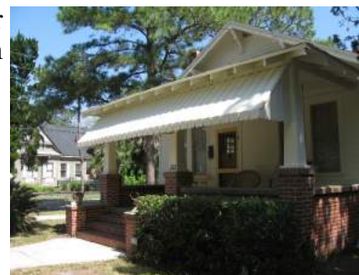
Example of appropriate metal awning added over a front porch.
