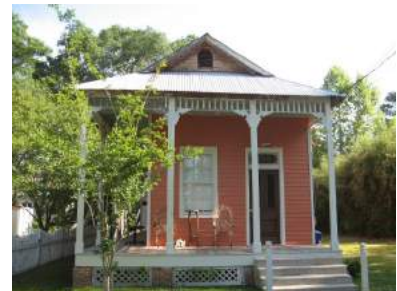
The dwelling at 22155 Main Street is an example of the “North Shore” or “Abita Springs” variation of a Shotgun plan.
