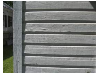
Example of original drop siding at 22119 North Street.
