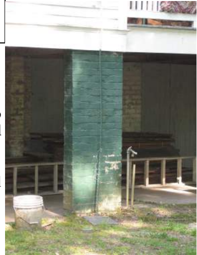
Brick pier foundation at 22166 Grover Street.
