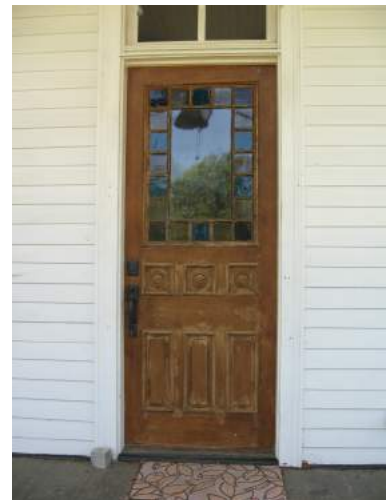
This decorative door at 71618 Maple Street has a large central light bordered by smaller color-tinted lights and a series of three square panels over three vertical, rectangular panels.
