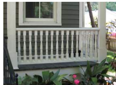
Original porch railing at 72170 Gum Street.
