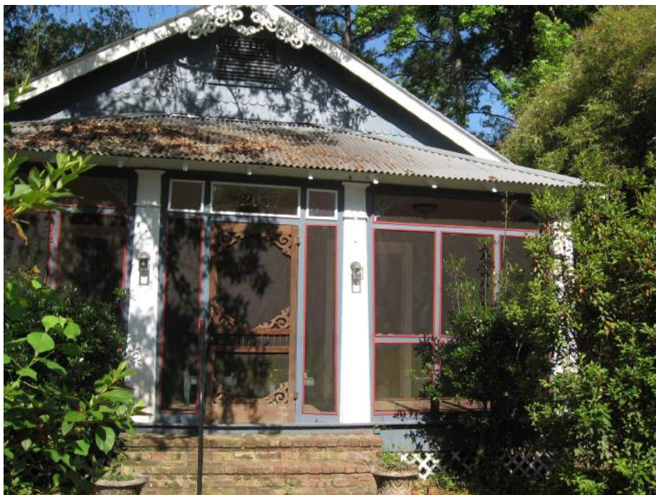
This porch at 72037 Laurel Street is appropriately screened, with sections inserted within the openings between its columns.
