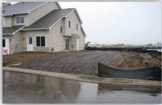
Properly constructed BMP for vehicle tracking.
