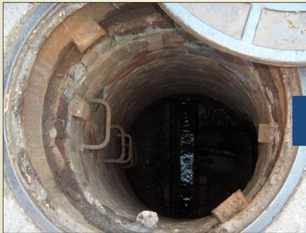
Typical Sanitary Manhole
